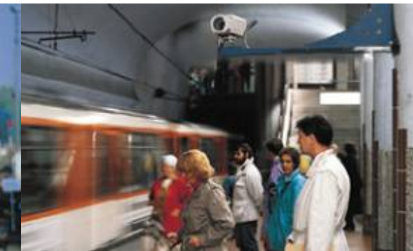
Telecommunications systems for rail applications
