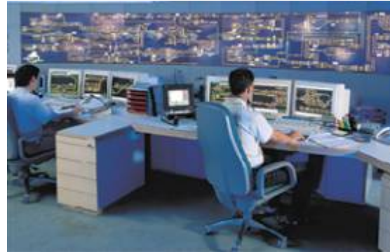
Interlockings and operations control systems
